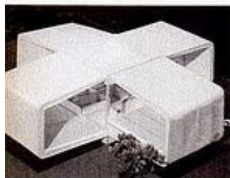
FIRST MODEL of plastic house shows the four U-shaped wings cantilevered out from a small central foundation. Actual test house, scheduled for '57, will follow a similar design.
